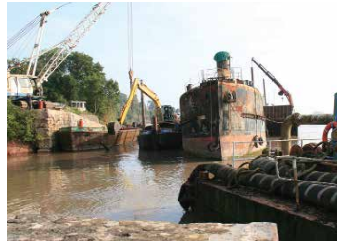
SS Freshspring is readied for turning and pushing into the Pill.
