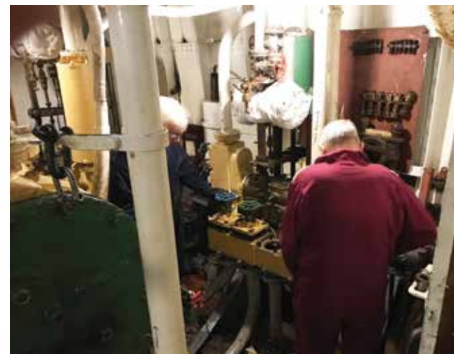
Work in the engine room in March 2019. Brian Gooding
