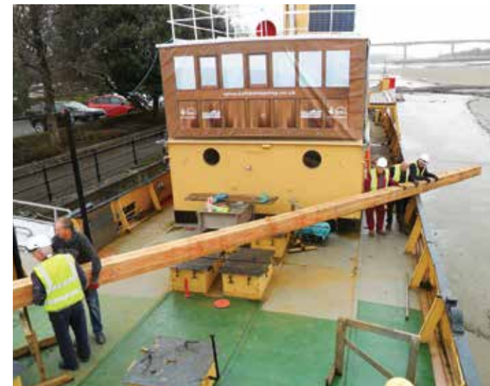
Manoeuvring the squared tree aboard ready for work to convert it to a new mast.
