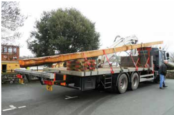
Arrival of the new mast.
