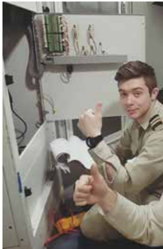
Fault finding on an AC unit.
