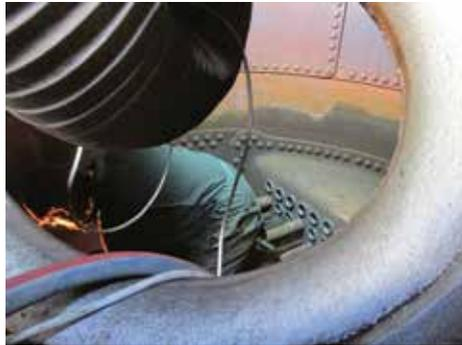
*Removing the flue tubes by cutting through inside the boiler.*
