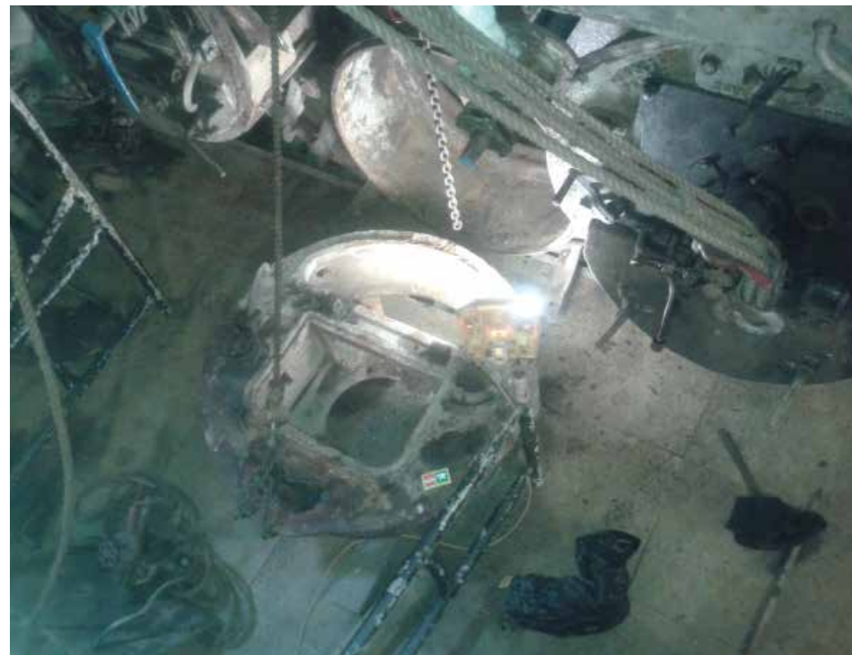
Furnace frontage safely down on the deck
