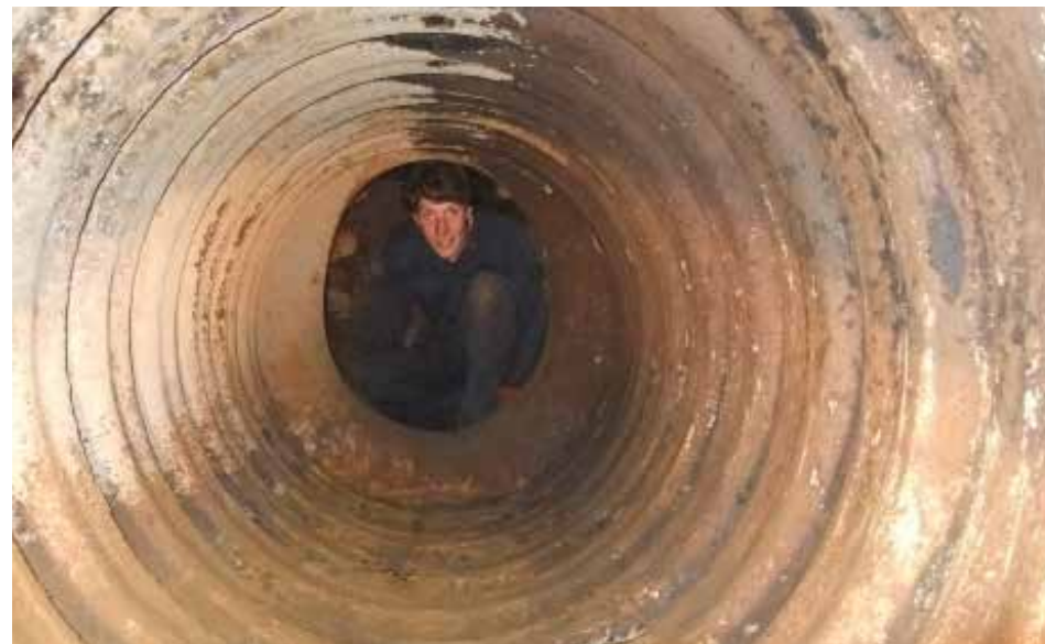
Mark Rozelaar scraping off the loose debris inside a furnace tube.
