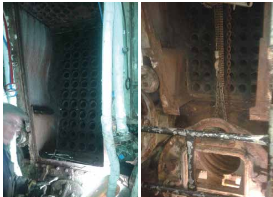
Alan Freebury unbolts one of the forced draft access panels.
