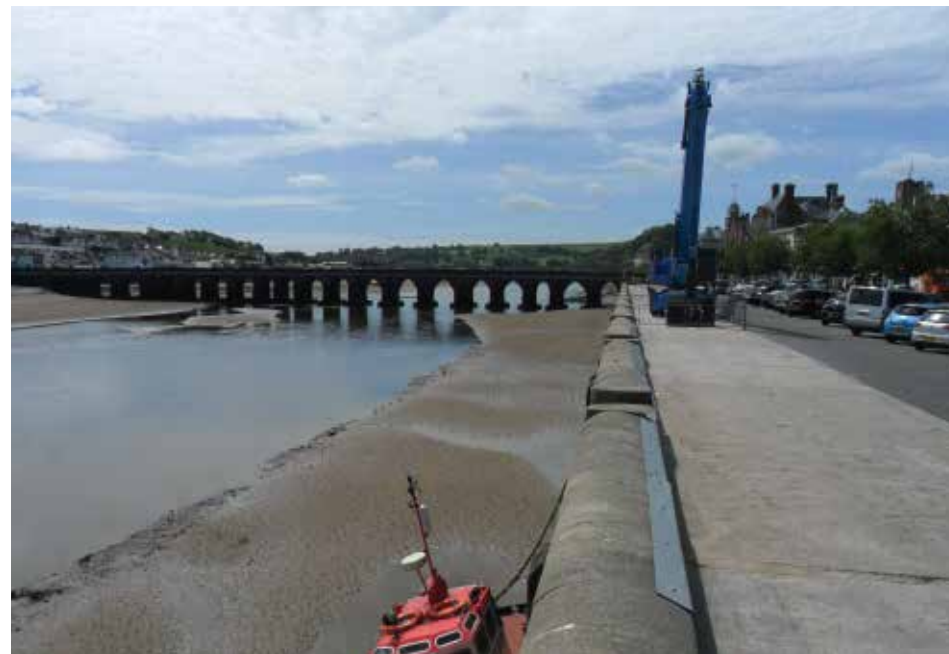
Looking south towards the town bridge. . .
