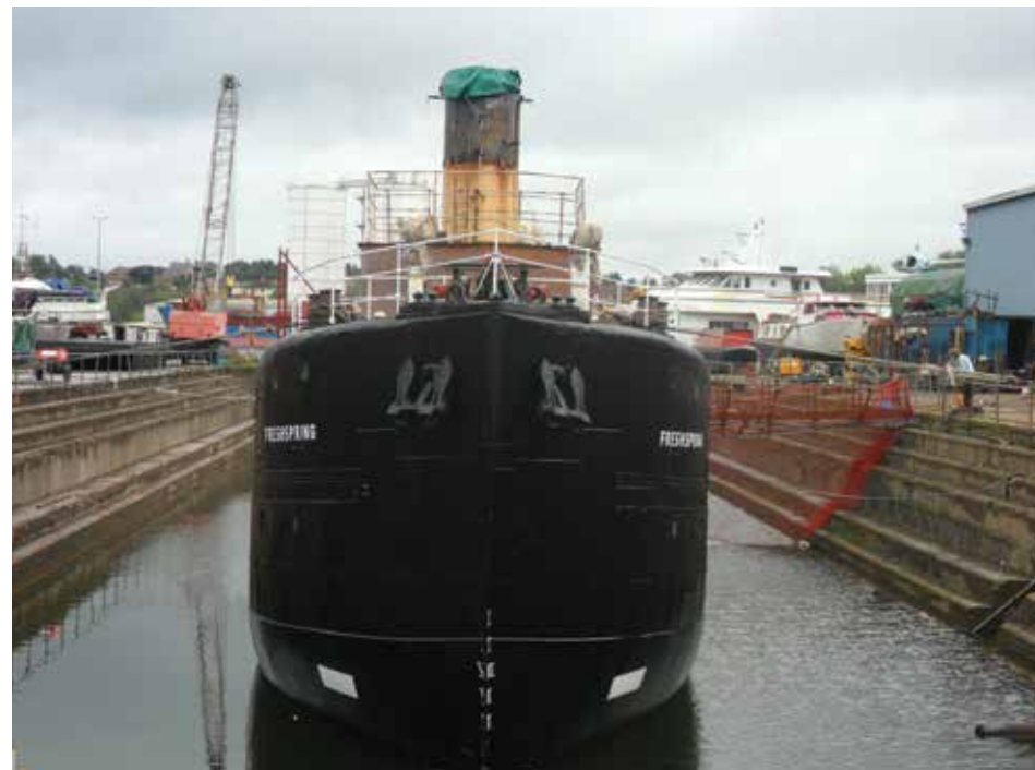
ABOVE: The drydock at Sharpness is filled to refloat Freshspring.
