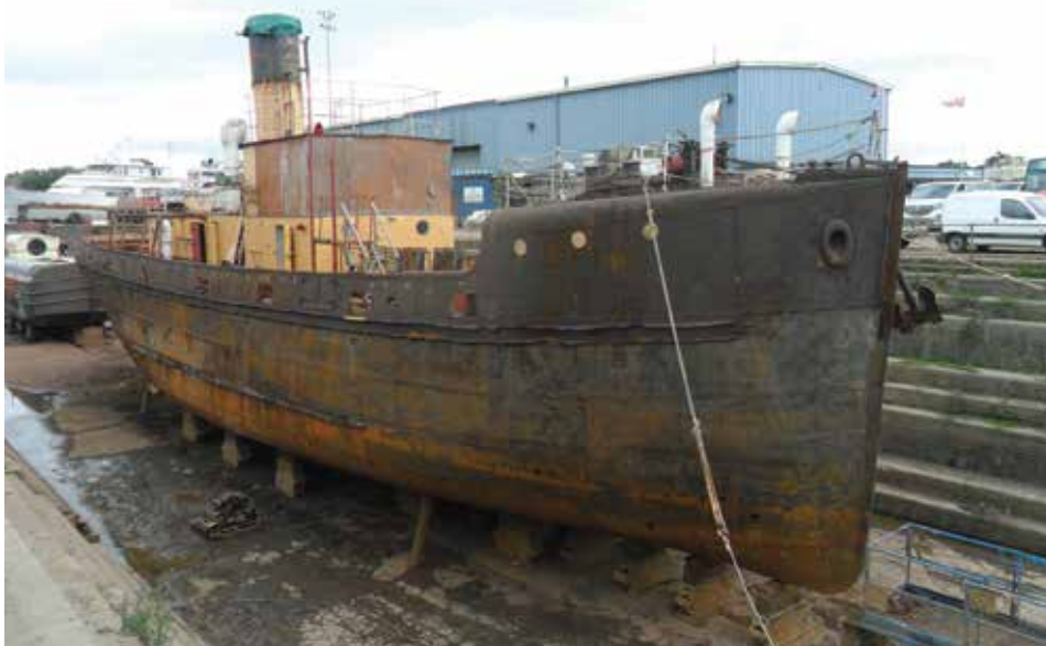
The hull has been cleaner prior to plating work starting.
