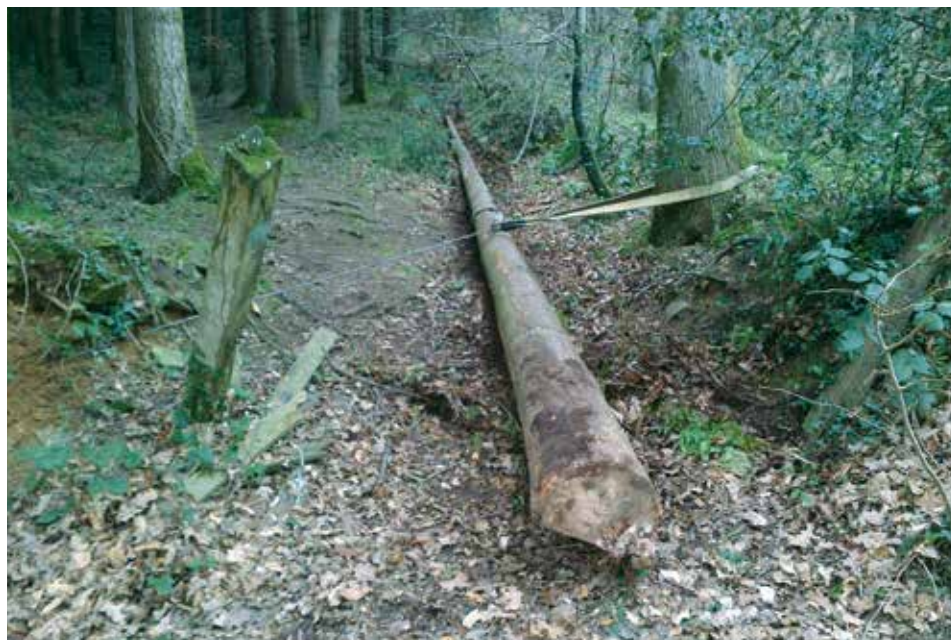
The tree for the mast is winched out of the woods. JP
