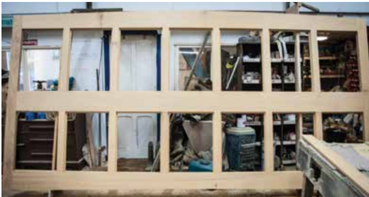
The front wheelhouse side with the rails and stiles all assembled.
