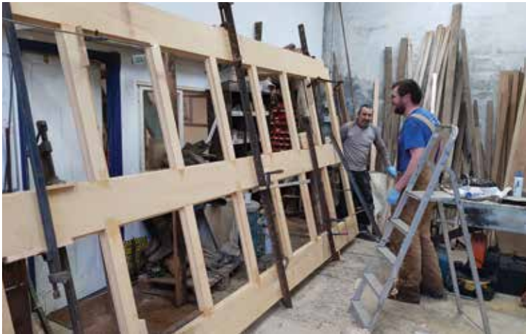
Keith and Chris assembling the wheelhouse front.
