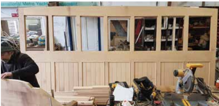
The front wheelhouse side with the panelling in place.
