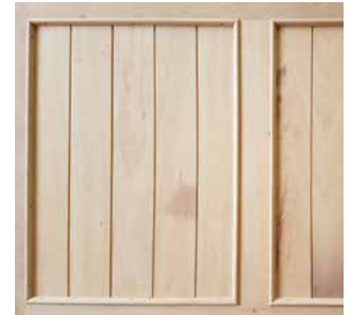
Detail of the lower panels. These are bedded on brown Sikaflex and held in position by the panel beading. The grooves and end grain for the panels was oiled prior to assembly to minimise water ingress.
