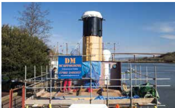
With the old plywood removed, the next step was to prepare the base for the new wheelhouse.
