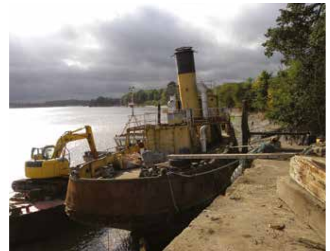
Brian's first view of the ship at Newnham back in October 2010. Note the access – a scaffold board on a ladder, balanced on a tyre and some pallets!
