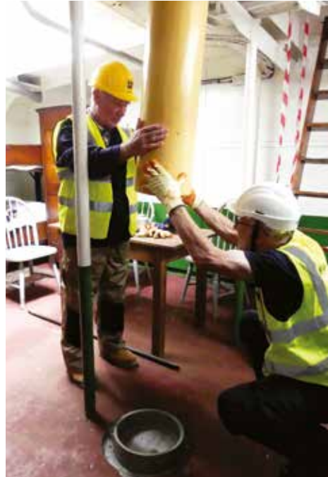
Lowering the mast into place in the forwards accommodation. Graham Hobbs
