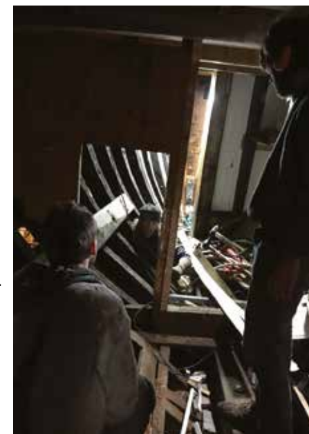
Work going on deep in the vessel.
