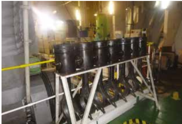
Generator pistons removed.
