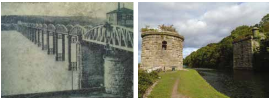
The Severn Rail Crossing before demolition (left) and the piers as they are today on each side of the canal (right).
