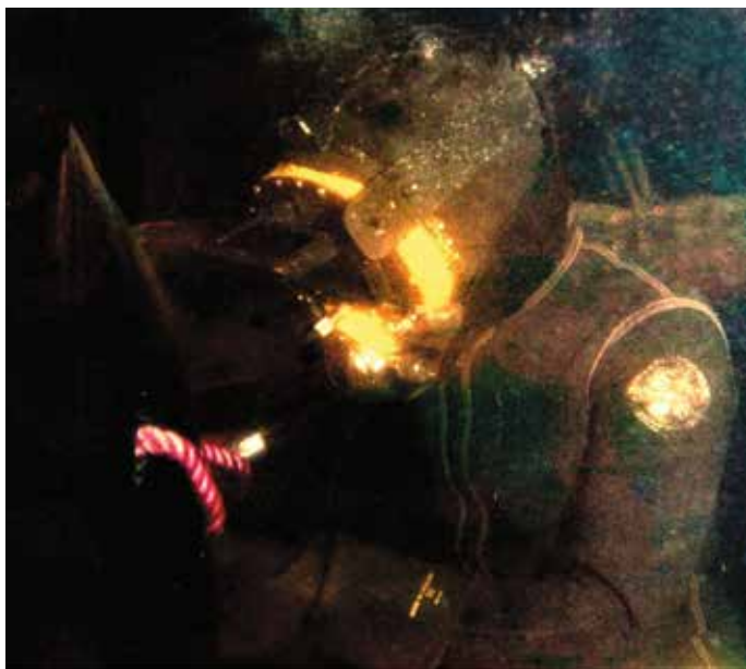
Kevin preparing to weld repairs to the hull.
