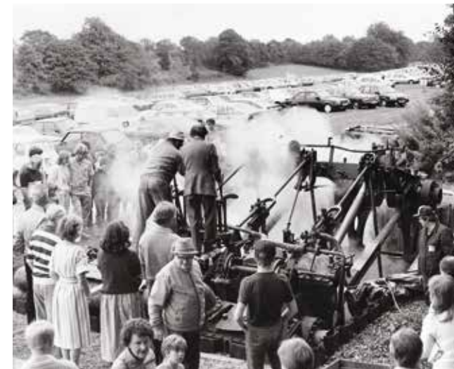
The engine of the Caledonia being run at Hollycombe for the first time. Cdr Baldock is on the right on the driving platform.
