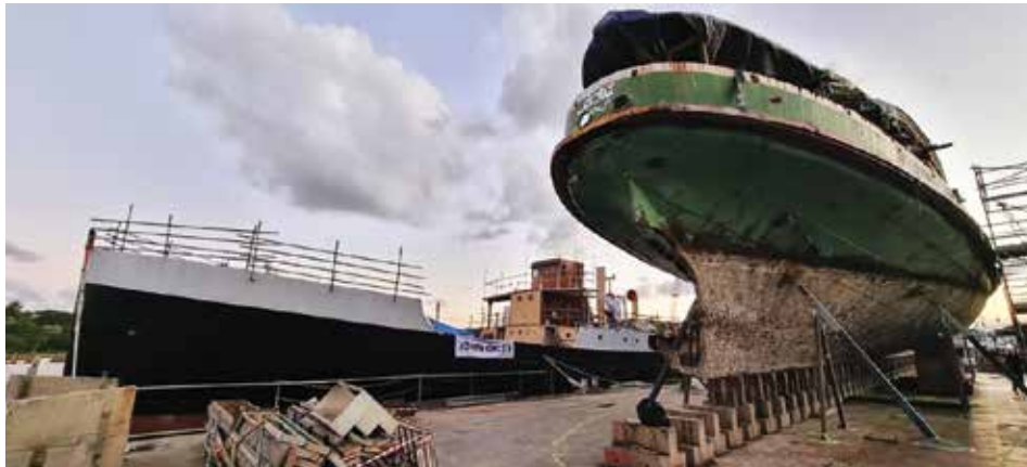
The Fleet's shipyard and two current restoration projects; Pilot Vessel John Oxley (1927) and Sydney Harbour ferry Kanangra (1912).
