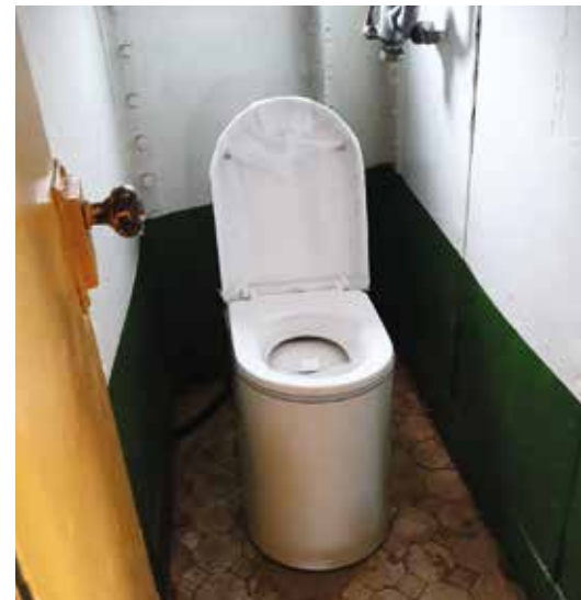
The new compostion toilet on the ship.
