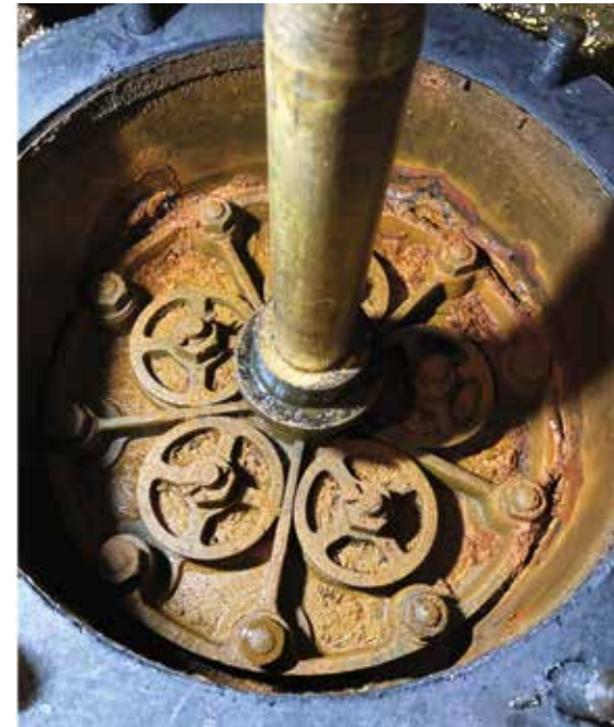
Upper chamber and valve cover plate before cleaning.
