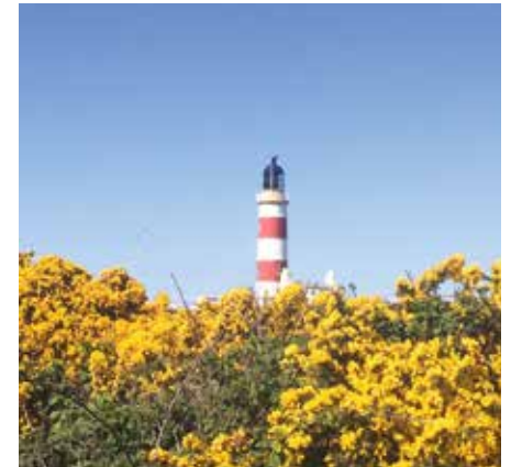
Point of Ayre lighthouse on the Isle of Man, red and white striped for easier identification in daylight.
