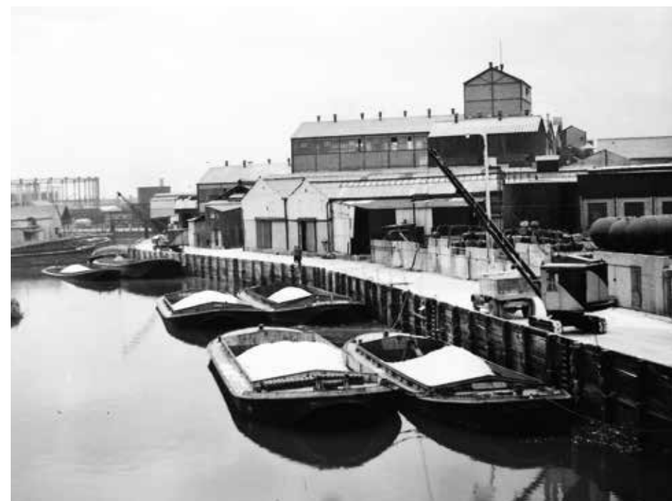
Unloading sand or similar material from lighters with grab fitted mobile cranes on the River Lea, 1950s. Reg Batten
